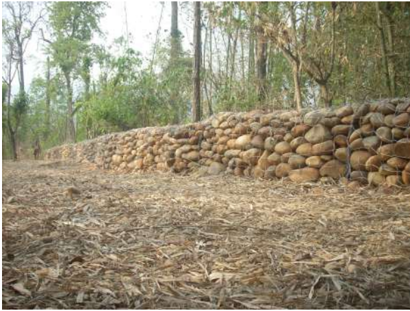
Photo: construction of gabion wall
