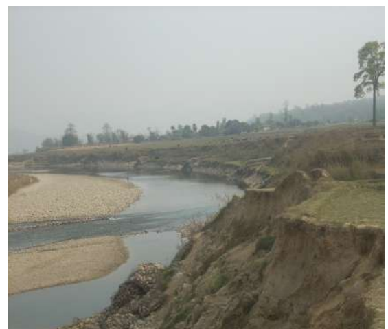
Photo 9: Vulnerable 186 HHs of Tandi-2 in the bank of Kamala River
