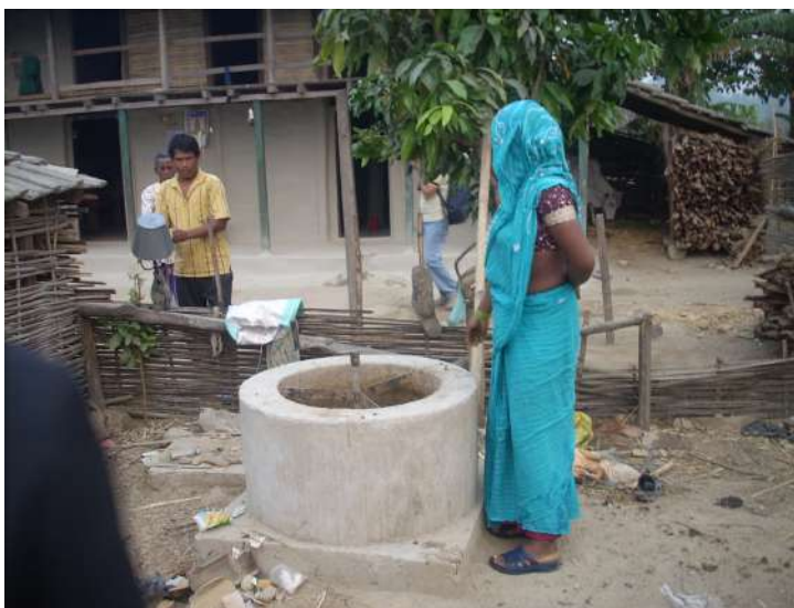
Photo : Bio gas plant establishment.
