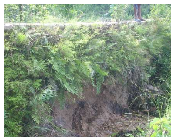
Photo 5a : Tandi irrigation canal prior to construction
