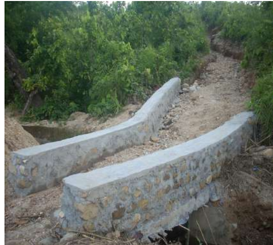
Photo 5c: Tandi irrigation canal after support
