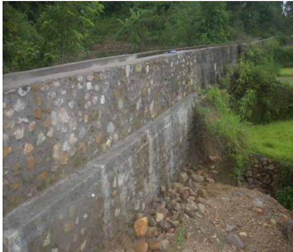
Photo 5b: Tandi irrigation canal after support
