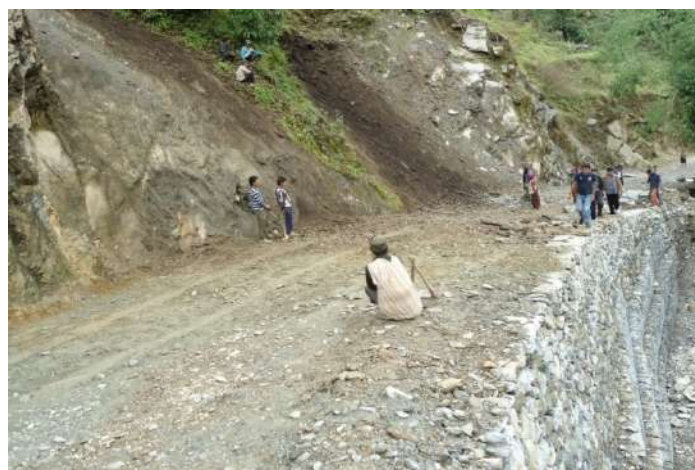
Road construction in Pyuthan
