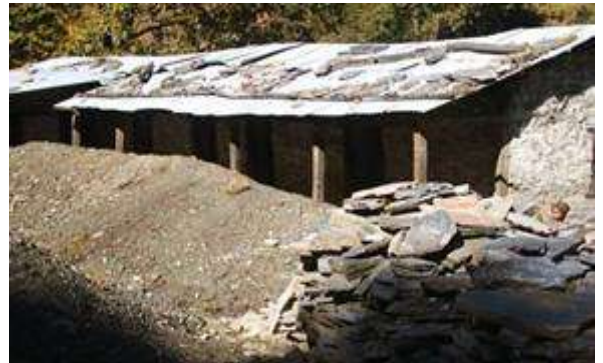
Gyanodaya P.S, before construction
