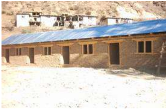
Gyanodaya P.S. during construction
