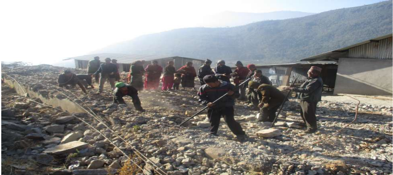
Beneficiaries working in debris clearance work
