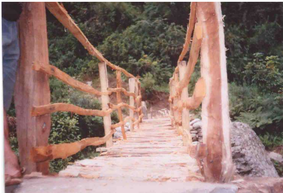
Photo 7: Wooden bridge in Dhime VDC, Jajarkot
