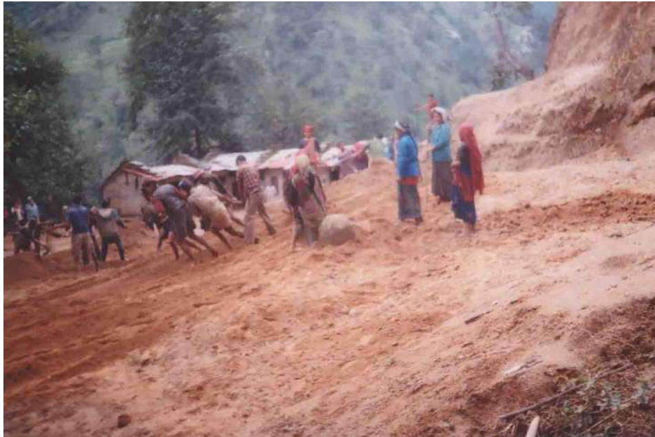
Photo 6: Workers busy in construction of School playground in Daha VDC
