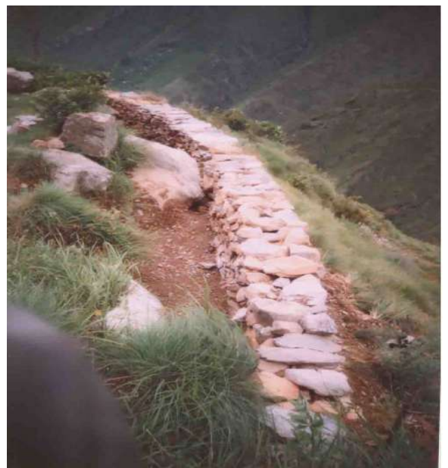
Photo 5: Laxmi PS boundary wall construction, Bhagawati VDC-9
